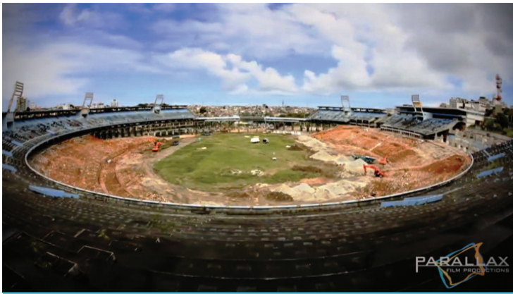
The demolition of Fonte Nova Stadium, Brazil
